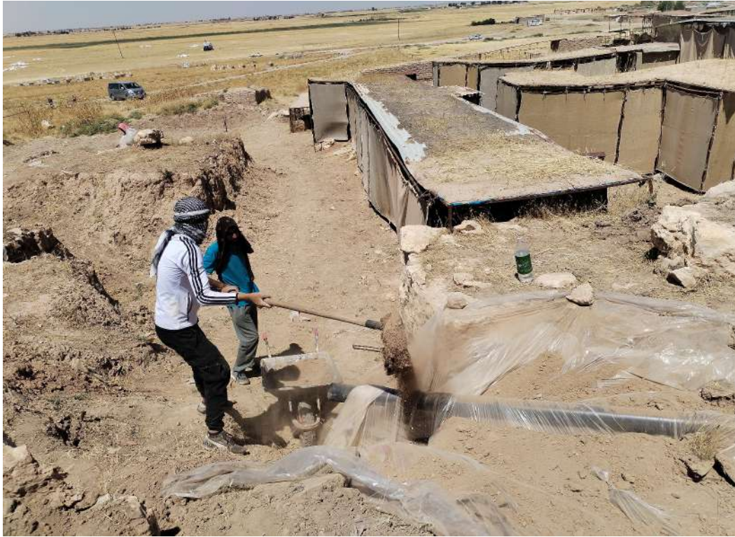
Fig. 11: Pit Backfilling
